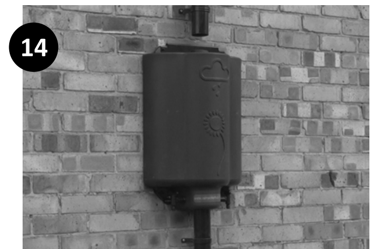
14. Attach hose connectors, and insert filter. The installation is now complete.
