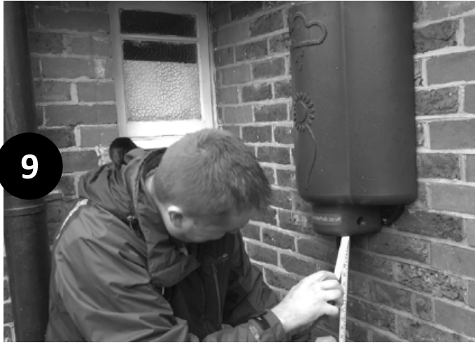
9. Measure and cut the lower section of downspout.
