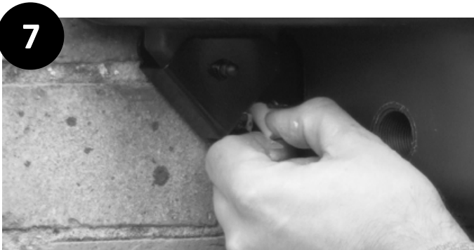
7. Re-hang RWH and mark drill holes for bottom bracket. REMOVE RWH and drill pilot holes (wood siding) or holes for masonry wall plugs.
