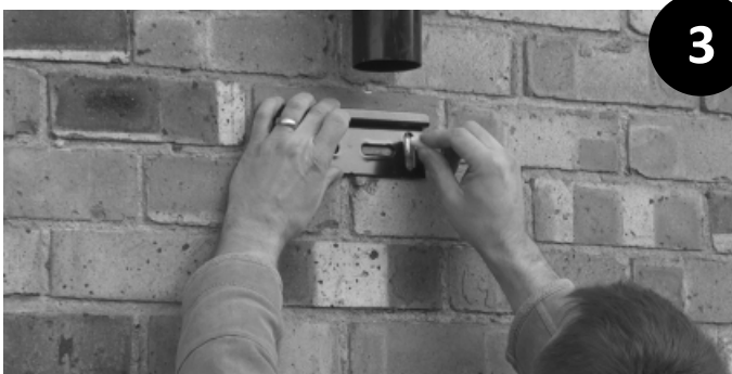
3. Position the top bracket 1" below the downspout and mark the holes to be drilled in the VERTICAL SLOTS using the pencil provided.
