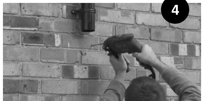
4. Drill in the centre of the pencil lines and insert the wall plugs (masonry wall).
