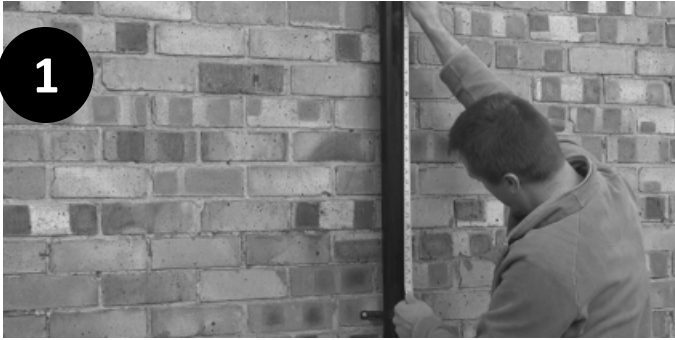
1. Measure a 27 1/2" length of downspout and remove.
