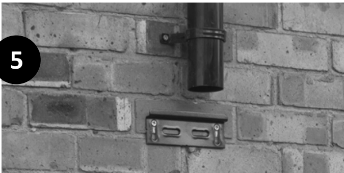
5. Through the VERTICAL SLOTS . Attach to the wall with wall plugs and COUNTERSUNK screws. Do not fully tighten yet.
