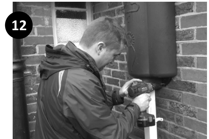
12. Now secure the lower bracket of the RWH using the two round-head or domed screws.
