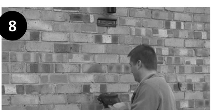
8. Insert wall plugs if used. Re-hang RWH. Do not screw in lower bracket yet.
