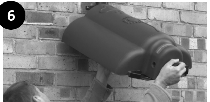
6. Holding the RWH at slightly less than 90 degrees, clip top bracket of RWH onto the mounting bracket on wall. Allow RWH to pivot down so that is flush with wall. Check alignment and adjust if necessary. Remove RWH tighten top screws fully.
