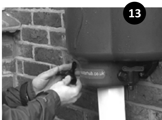
13. Screw in faucets with o-rings. Ensure secure and tight fit, but do not over-tighten.
