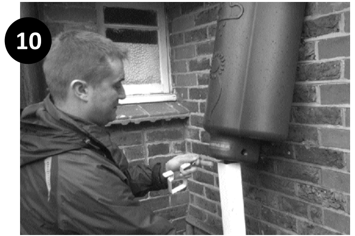
10. Insert RWH into downspout by angling both forward until they meet and then lowering them back together until flush with wall.
