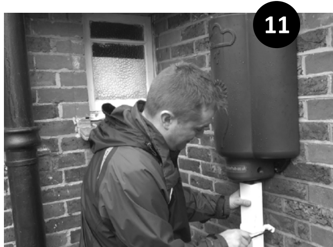
11. Re-fit lower downspout section.
